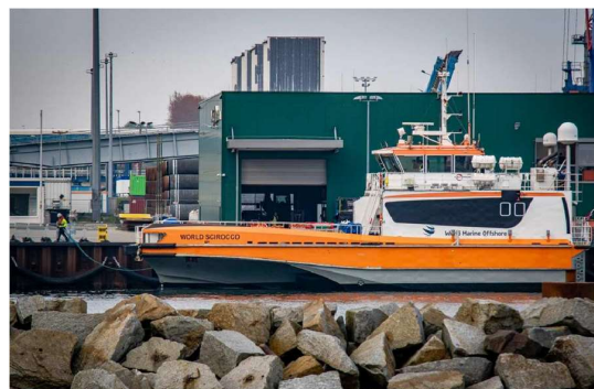
Photo 1. Operation Center and warehouse of Iberdrola with CTV in Sassnitz (Germany) (photo: Van Oord)
